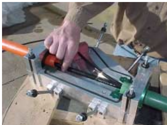
Figure 10 Hand Push Cable into Y-Block
