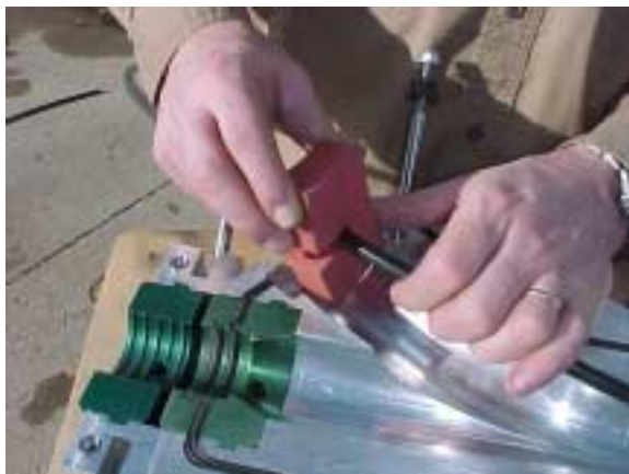
Figure 8 Install Cable Seal
